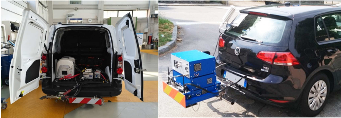
Figure 1. Installation of PEMS main units left) inside the vehicle right) outside the vehicle
